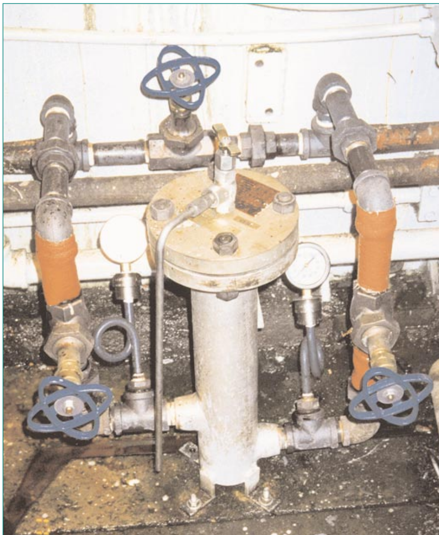
Photo 2. The HTF filter in a sidestream installation. The inlet of the filter is installed close to the pump's discharge. Fluid is diverted through the filter, cleaned and discharged to the suction side of the same pump, or to a low-pressure return line.
